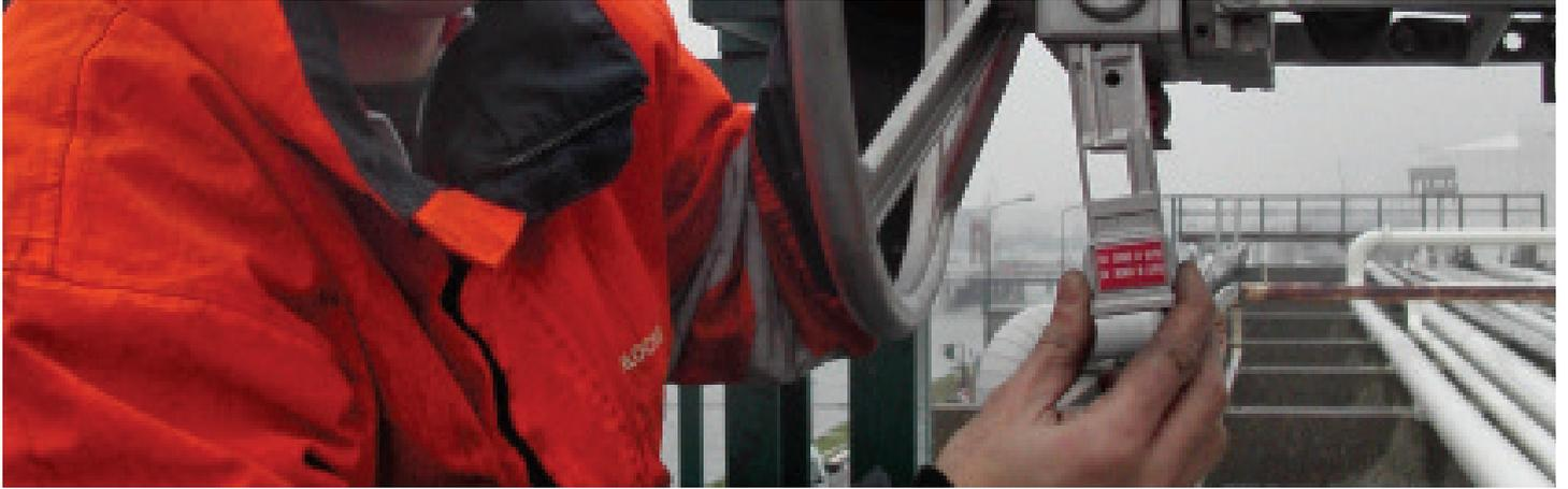
the total removal of the interlocks from the valves. An experienced valve interlock service engineer has extensive experience in reading and understanding interlocking sequences. He is trained to understand the sequence path from a LOIS and translate that to the situation in the field. Third party installation teams should receive proper training on reading sequences prior to their installation job.
