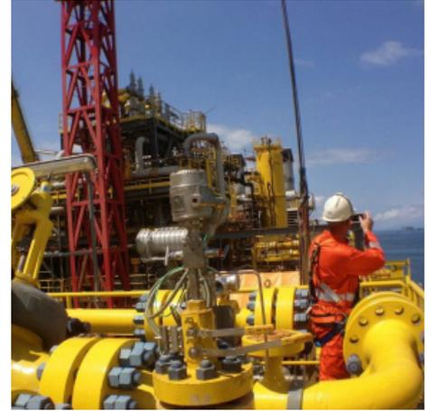
A valve interlock is added on top of a valve to ensure that the valve can only be operated in a predefined sequence with the other valves of the same system. For standard interlocks, installation is done by bolting only. Any type of hot work or amendments to the host valve is not required. The mounting of an interlock to a valve is not complicated. Therefore many users and contractors choose to install the interlocks themselves.
