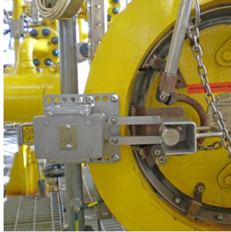
During pig launching and receiving, operating procedures must be followed carefully. When the vessel is not drained and vented or when the isolation valves are not fully closed before opening the closure door, very dangerous situations can occur. The Netherlocks Closure Lock (CL), as part of an interlocking sequence, prevents these situations by guaranteeing that the isolation valves are closed and the vessel is vented and drained before the closure door can be unlocked and opened.
